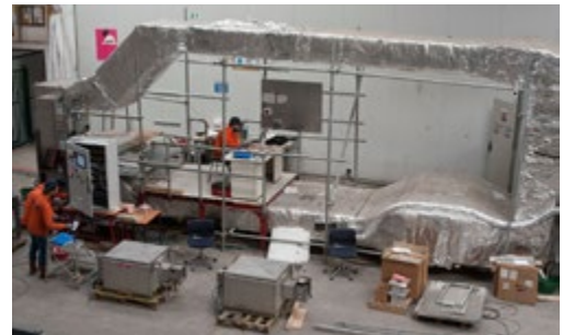
HVAC bench for FAT
