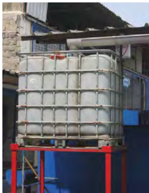
Water tank collecting rain water - Republic of Congo
